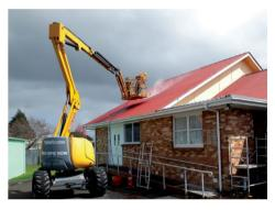
This project was to paint the exterior of the church and roof. With the Health and Safety requirements not allowing workers to be on the roof it was decided the best approach for this project was to use a cherry picker. This allowed James and Lejf to water blast and spray paint the roof without standing on it. Team Leader - James Pask, Glen Bavister, Anita Pedersen, Lejf Pedersen, Graham and Colleen Stokes and Mervyn Taylor.
